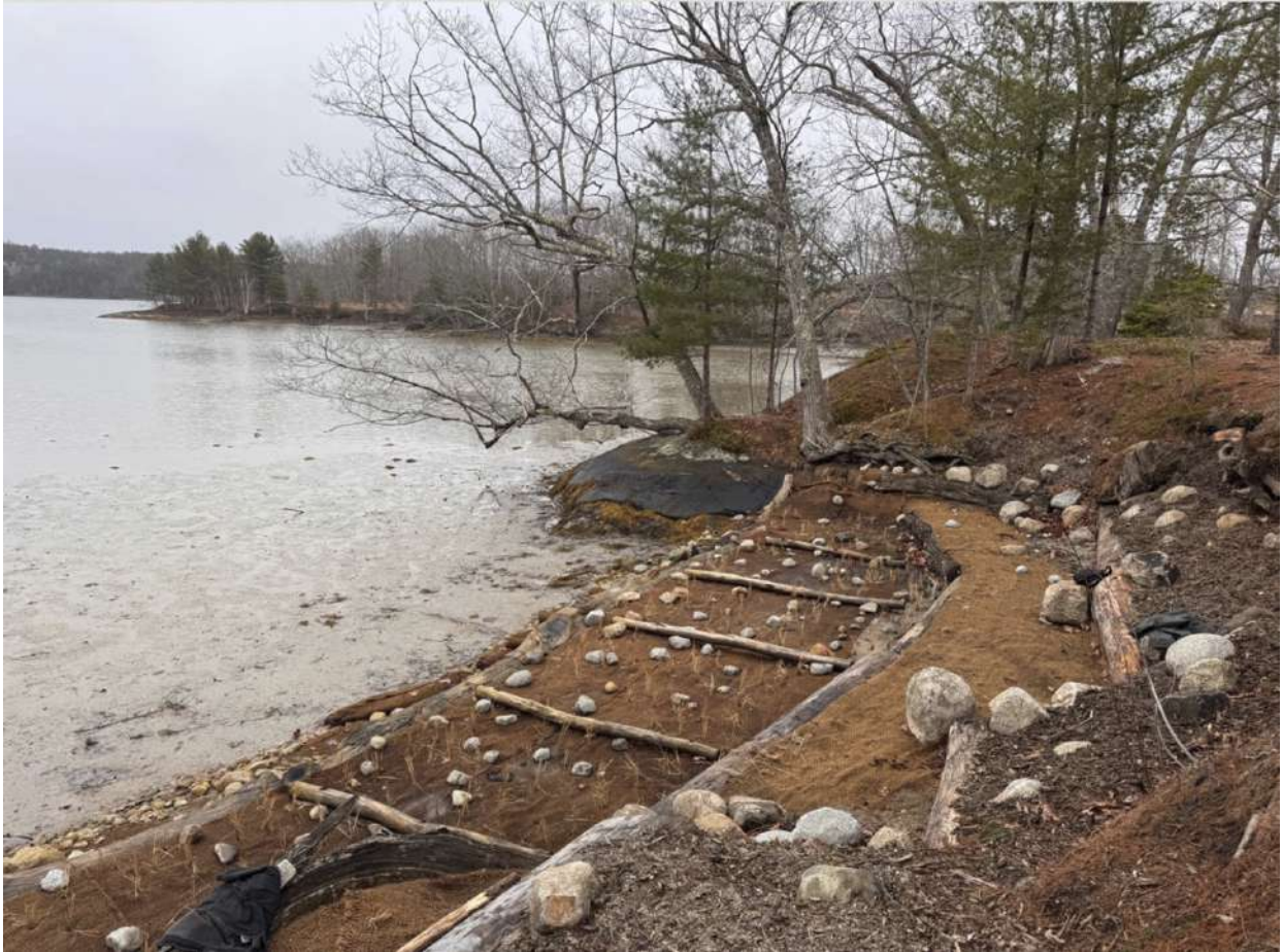
Figure 8: Example of a log sill installed for marsh restoration. (Photo from Treyball & Bernacki, 2025).
