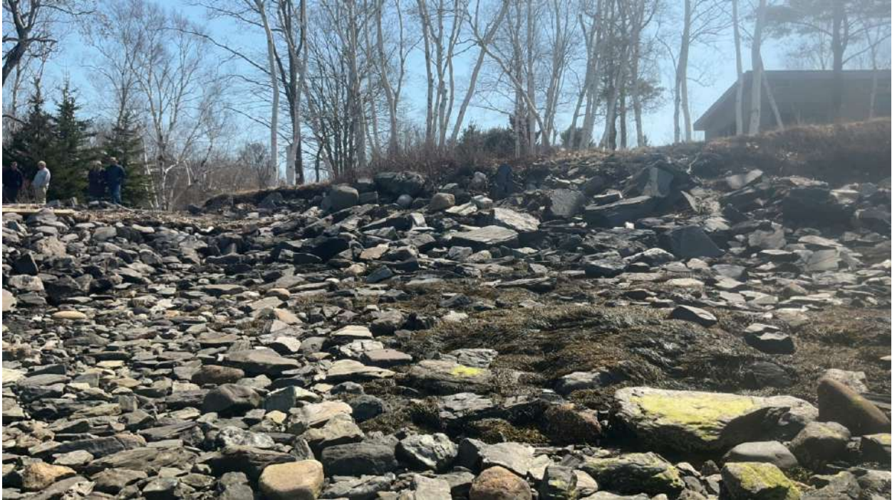
Figure 1: A section of the shoreline including the barge landing to the left.
